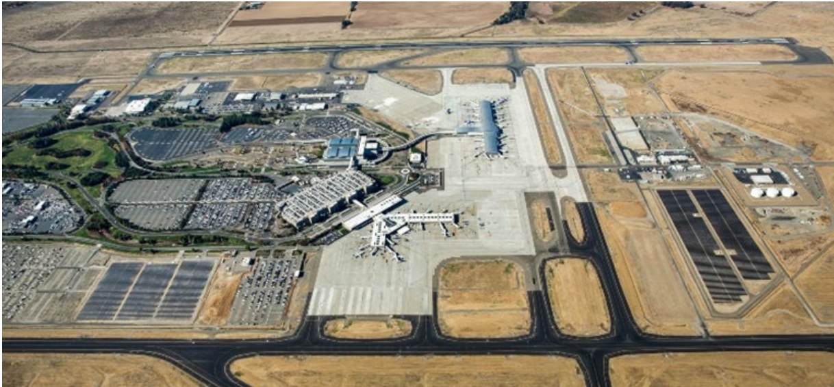
Figure 1-1 Solar Facilities at SMF
