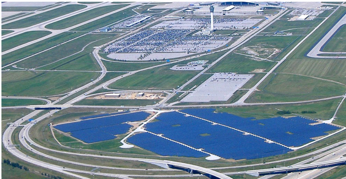
Figure 1-2 Solar Facilities at IND
