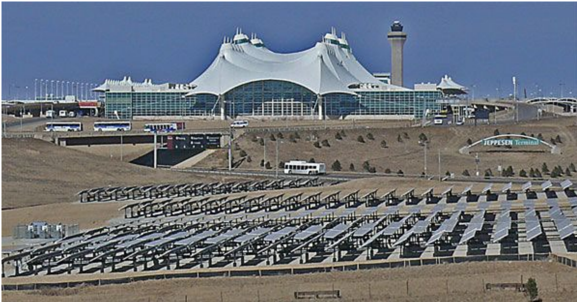
Figure 1-3 Solar Facilities at DEN
