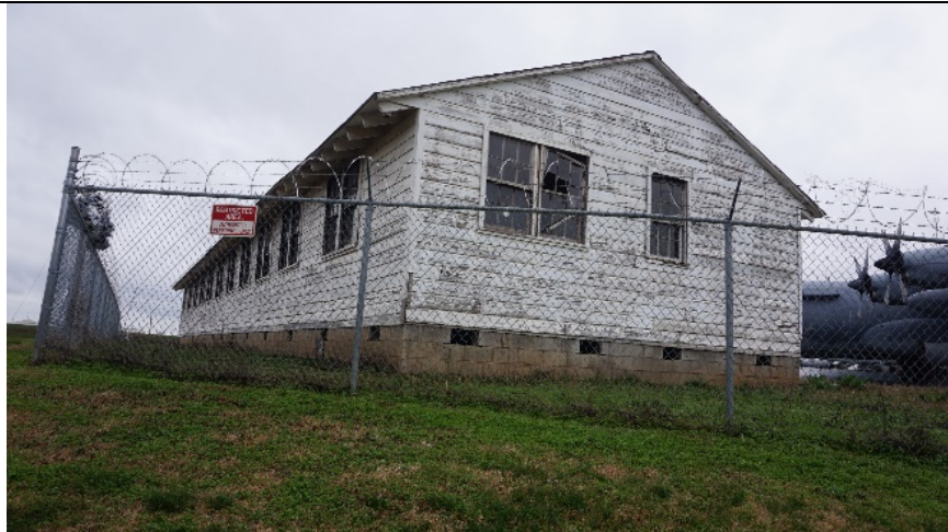
MK3825_ThomasW.FerebeeBuilding,ArmyAirCorpsMorrisFieldBarrac ks_02 20_V.W._03
