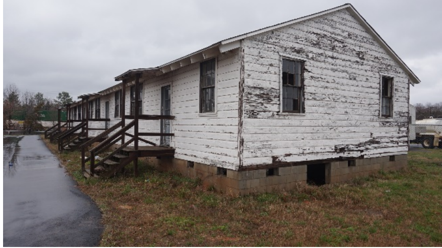
MK3825_ThomasW.FerebeeBuilding,ArmyAirCorpsMorrisFieldBarrac ks_02 20_V.W._01
