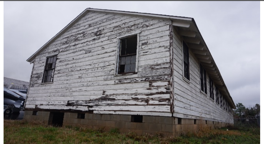
MK3825_ThomasW.FerebeeBuilding,ArmyAirCorpsMorrisFieldBarrac ks_02 20_V.W._04
