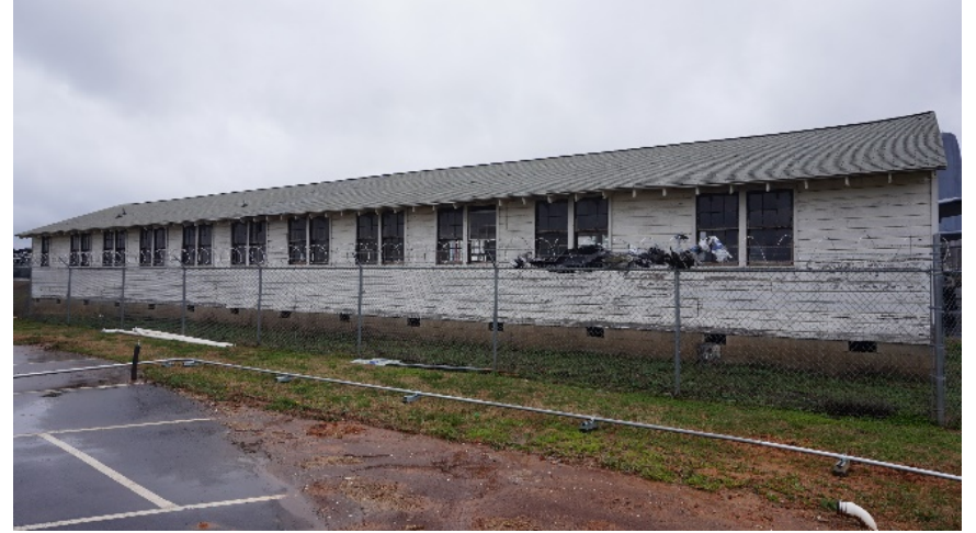
MK3825_ThomasW.FerebeeBuilding,ArmyAirCorpsMorrisFieldBarrac ks_02 20_V.W._02
